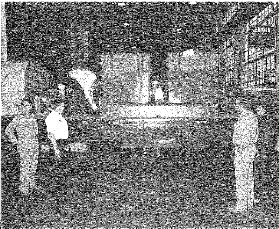
The repair of motor generators for Westinghouse Materials Company of Ohio required the involvement of most of the departments of the Maintenance Division. The third unit was loaded for shipment to Westinghouse April 27. The loading was observed by John Petry (D-711); Gene Wilburn, general foreman (D-711); Buzz Ison, foreman (D-711); and Kurt Lawton, project coordinator (D-742).
